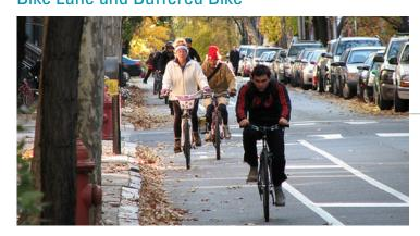
Bike lanes designate an exclusive space for bicyclists through the use of pavement markings and signage. Bike lanes are located adjacent to motor vehicle travel lanes and flow in the same direction as motor vehicle traffic. Buffered bike lanes are conventional bicycle lanes paired with a painted buffer space separating the bicycle lane from the adjacent motor vehicle travel lane and/or parking lane. These lanes provide greater separation between bicyclists and motor vehicles.
