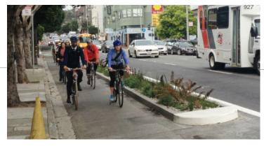
Separated bike lanes, sometimes called "cycle tracks" or "protected bike lanes" are dedicated bikeways that use a vertical element to provide separation from motor vehicle traffic. The vertical separation discourages drivers from parking or idling in the bikeway, and increases comfort for bicyclists. They are typically applied on roads with collector and arterial streets with high motor vehicle volumes, and moderate to high motor vehicle speeds.
