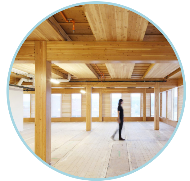
New cross-laminated timber floor mezzanine infill
