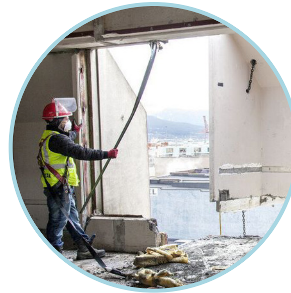
Demolish existing interior cells and pod walls
